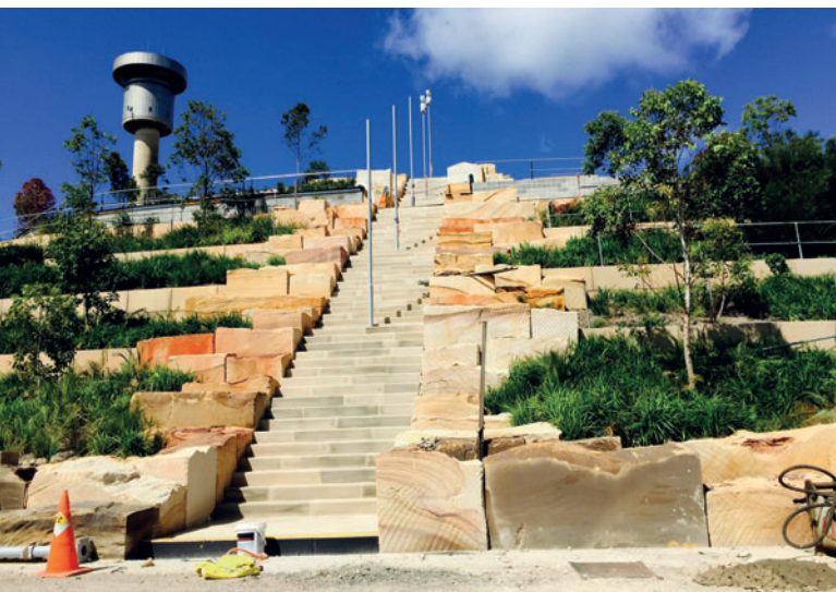
Austral Masonry colored the MagnumStone blocks to blend in with the sandstone blocks that rise from the shoreline and flank the stone staircase.
