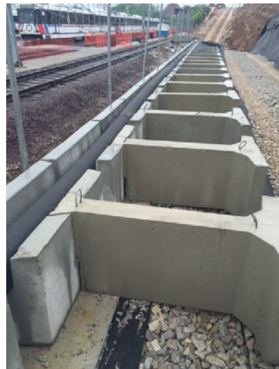
The tongue-and-groove extenders can be added in 2-foot increments, which provides stability that enables the gravity wall to be constructed to great heights.
