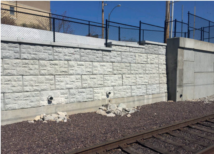
MagnumStone's hollow core design enables drainage features to be built into the system.
